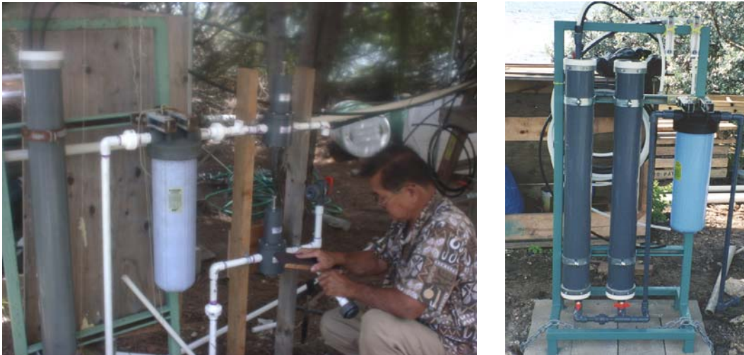
Figure 16. Installation of Pre-treatment and RO Units.
