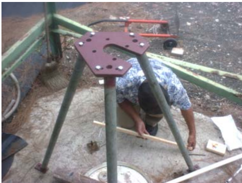
(a) Under construction
