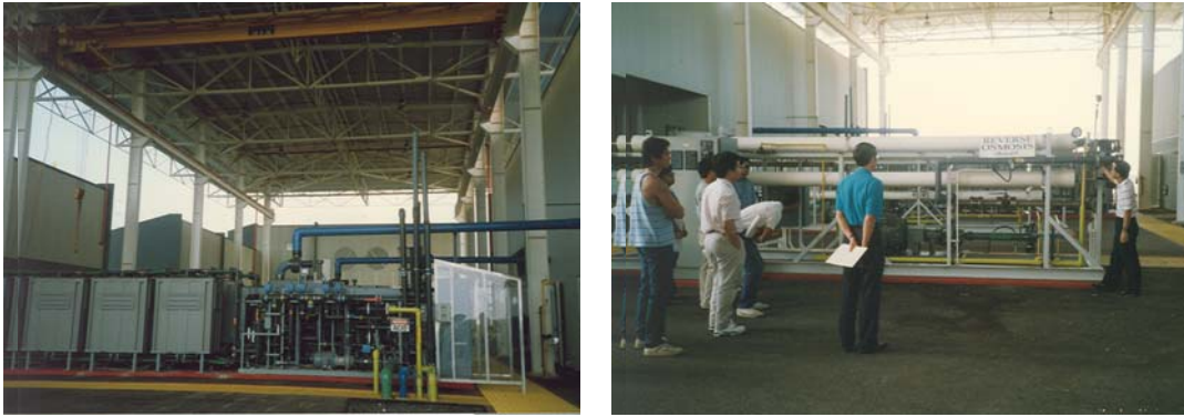
Figure 35. Existing State of Hawaii Demonstration Desalting Facility.
