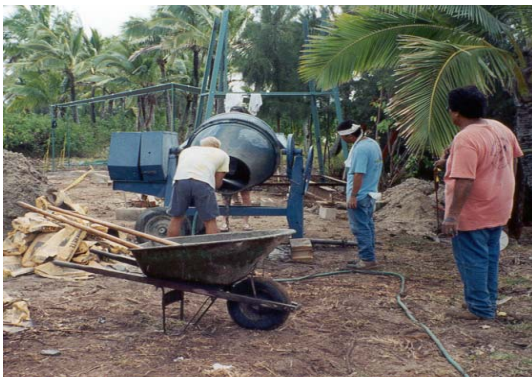
(a) Under construction
