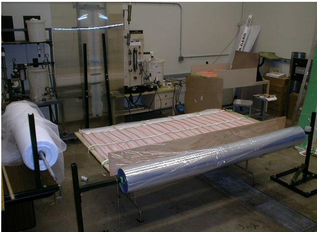
Figure 12.—Construction Start of the Heat Exchange Envelopes for the Pre-Pilot Unit.
