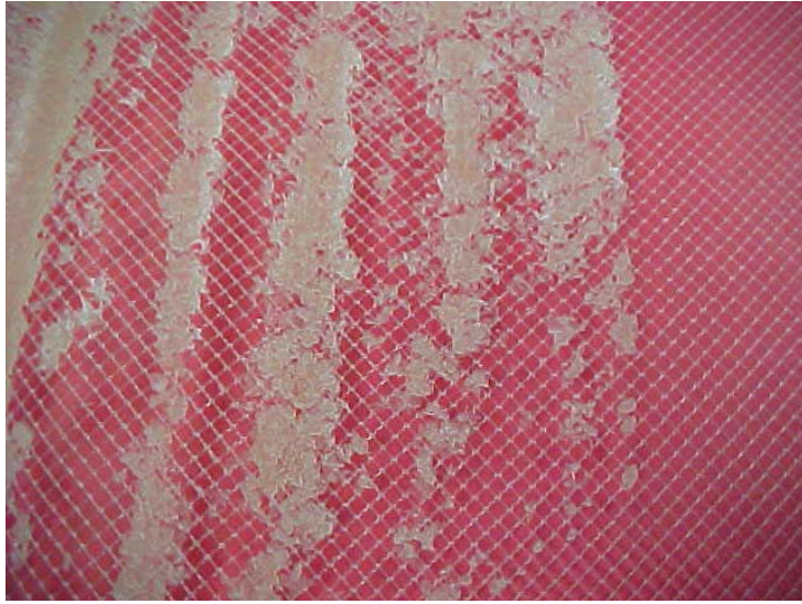
Photo 11.—Calcium Sulfate Scaling - HVC Installed on MU 1 Feed Tank.
