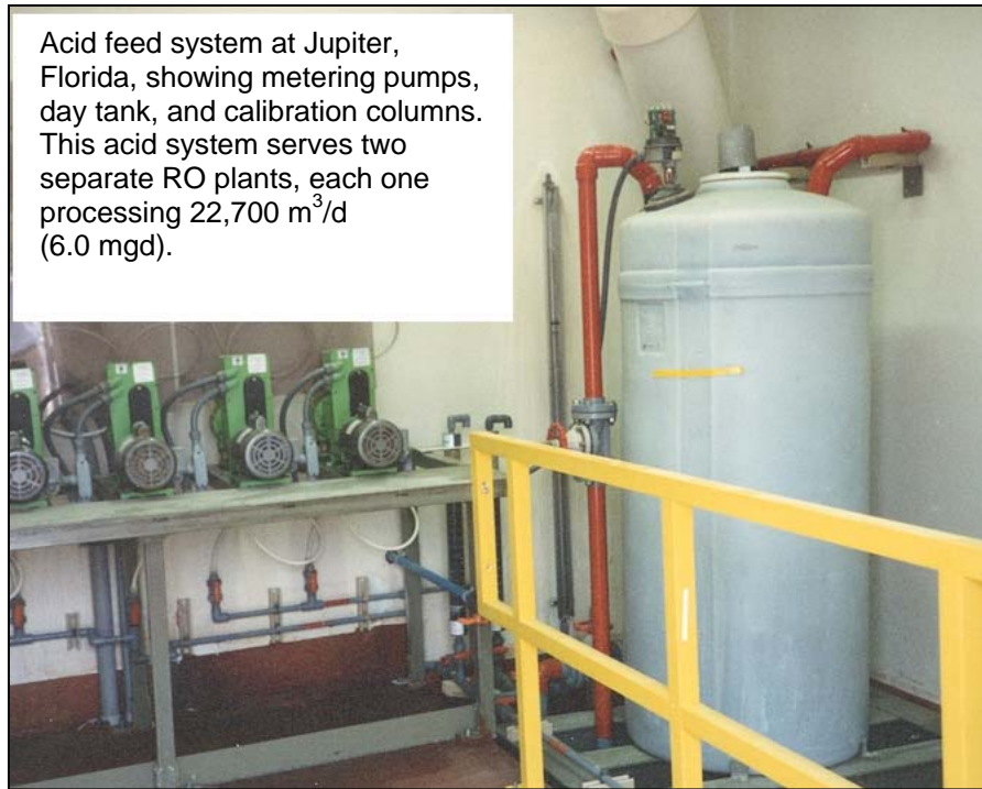
Figure 4-39 Typical chemical feed system
