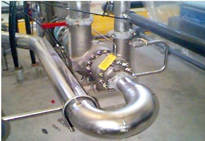
Small Pelton Wheel, serving two small SWRO units
