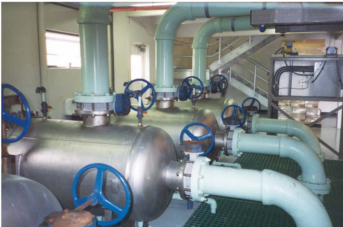
Figure 4-38 Horizontal cartridge filters in Jupiter, Florida
