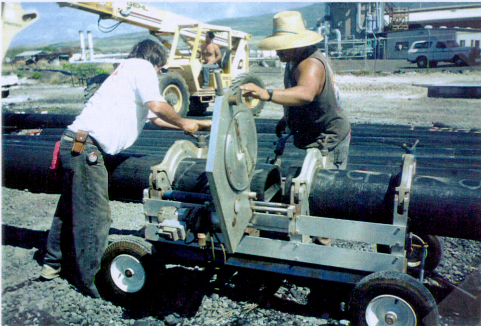
Figure 5-4: Thermal Welding High Density Polyethylene Shell Pipe
