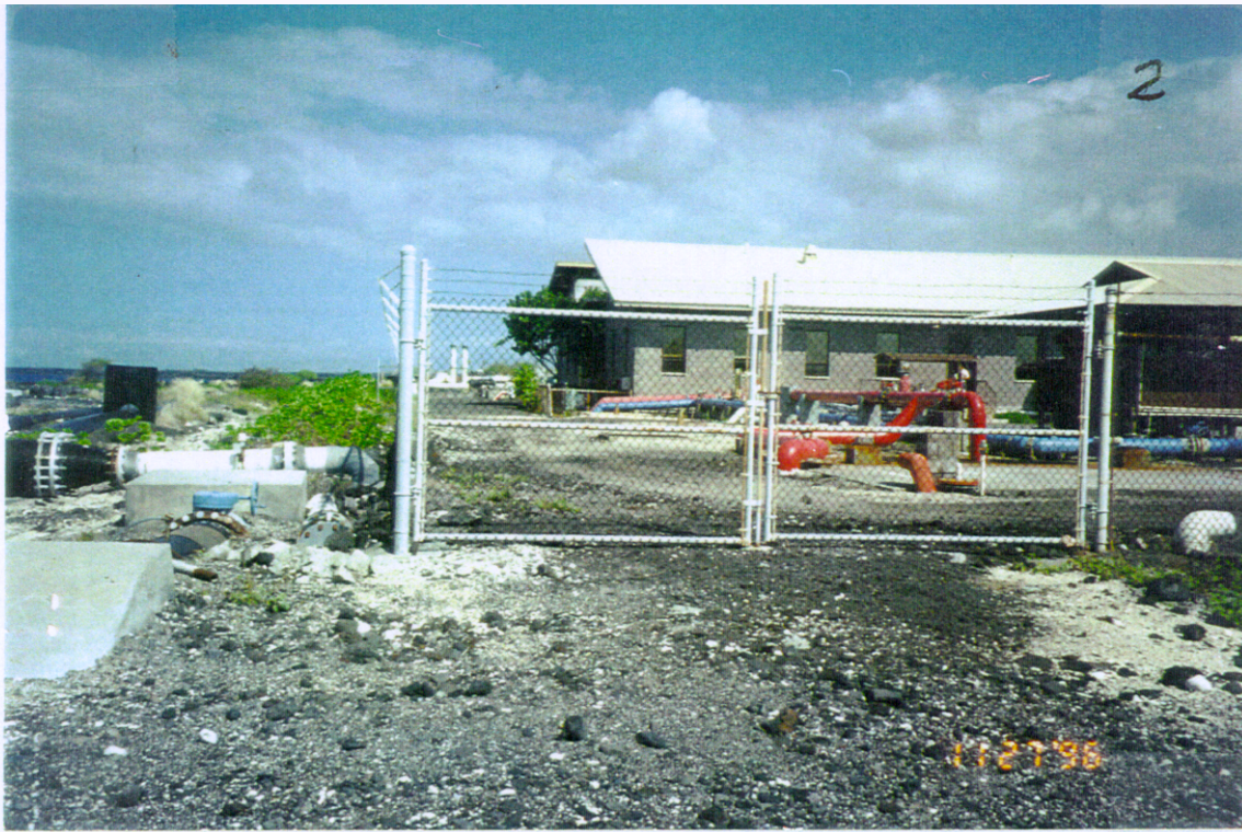
Figure 4-2: View North along NELH West fenceline
