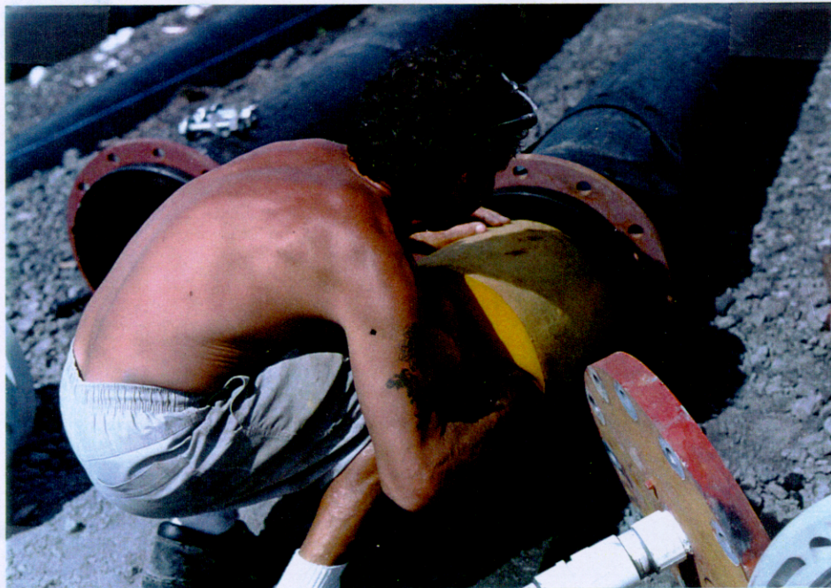
Figure 5-6: Shell Pipe Cleaning with “Pig”
