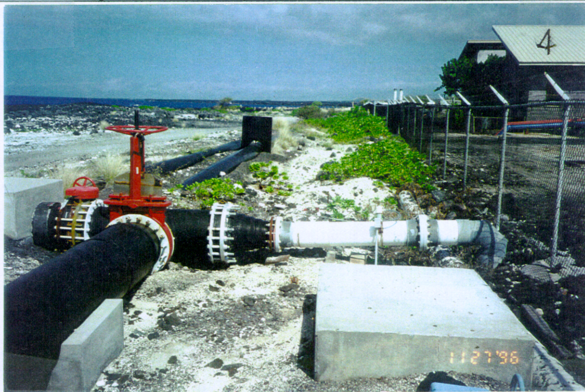
Figure 4-3: View of Crystallizer Laydown Area and Pedestal
