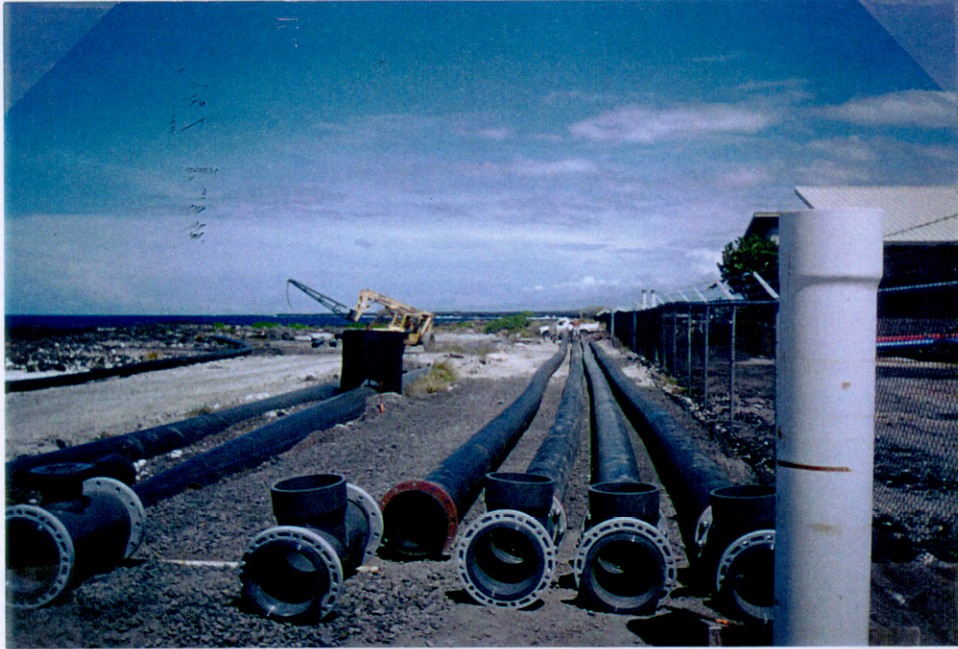
Figure 5-5: Crystallizer Shell Pipe Emplacement
