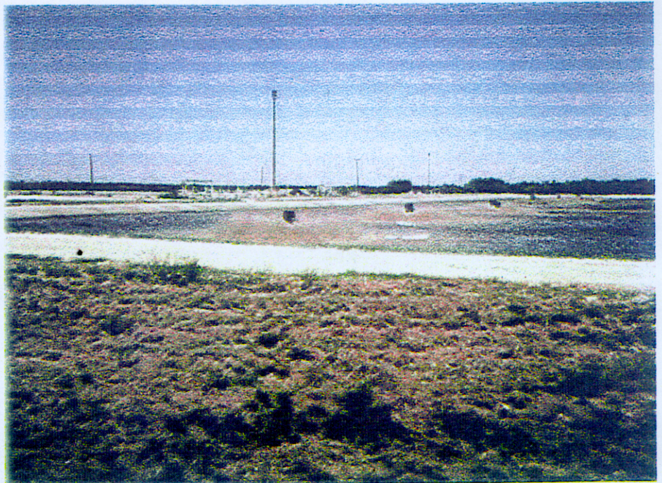
Exhibit A-8. Extended basins at McAllen WWTP.
