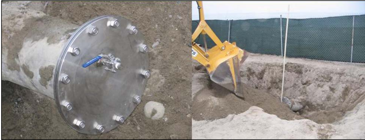
Below-ground completion of slant wells (photo by GEOSCIENCE).
