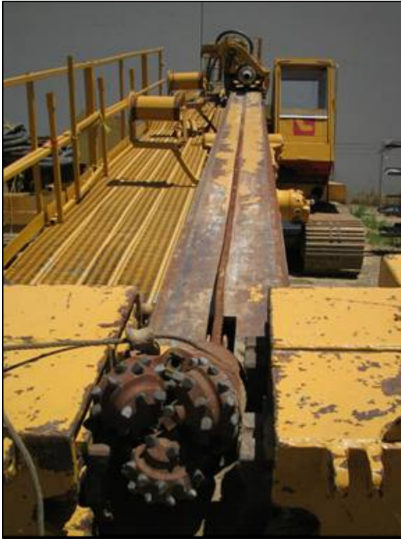
Cherrington HDD drilling rig (photo by GEOSCIENCE).
