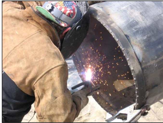
Welding carbide-studded guide shoe to casing (photo by GEOSCIENCE).
