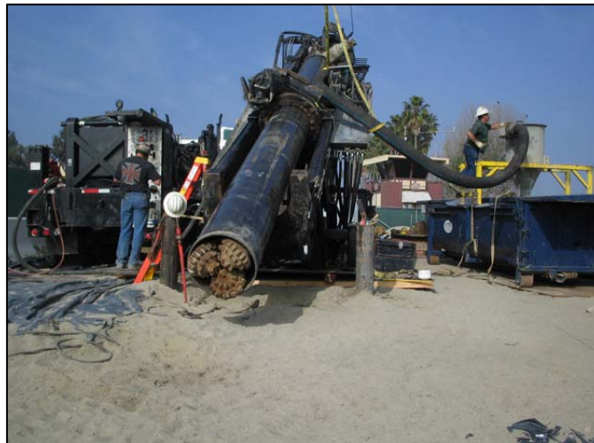
Starting to drill dual rotary test slant well (photo by GEOSCIENCE).
