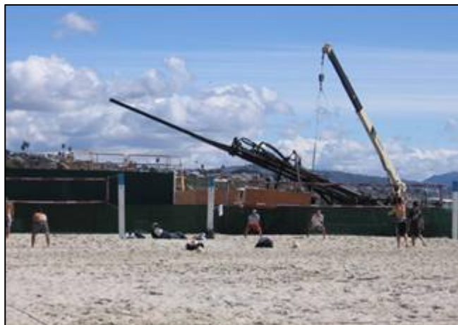
Slant well construction (photo by GEOSCIENCE).
