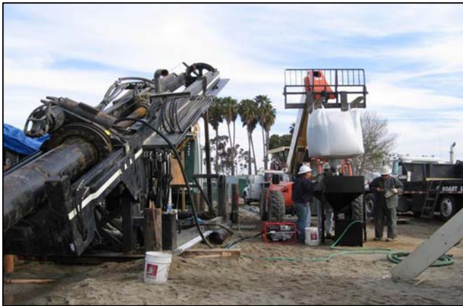
Gravel packing phase of slant well construction (photo by GEOSCIENCE).
