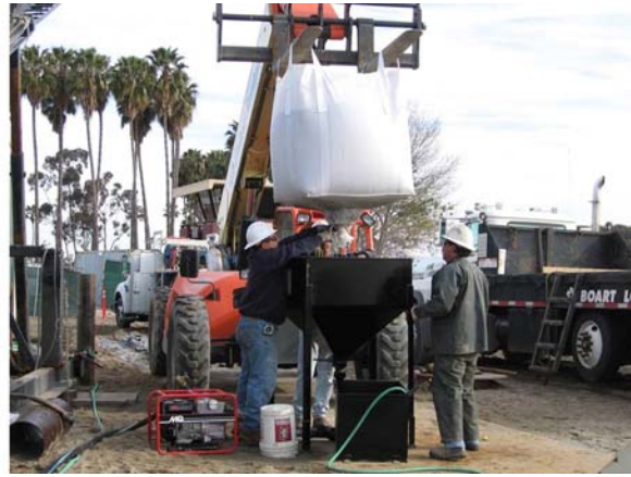
Filter packing the test slant well (photos by GEOSCIENCE).
