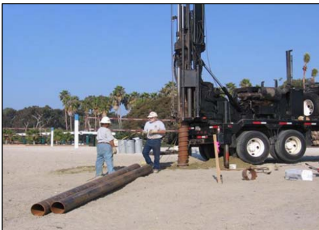
Drilling holes for anchor pipes (photo by GEOSCIENCE).
