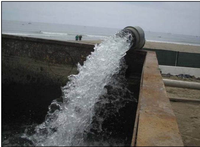
Discharging from SL-1 during pumping (photo by GEOSCIENCE).
