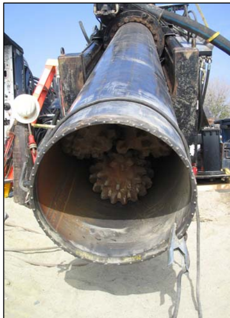
Dual rotary outer casing stabilizes borehole during drilling (photo by GEOSCIENCE).
