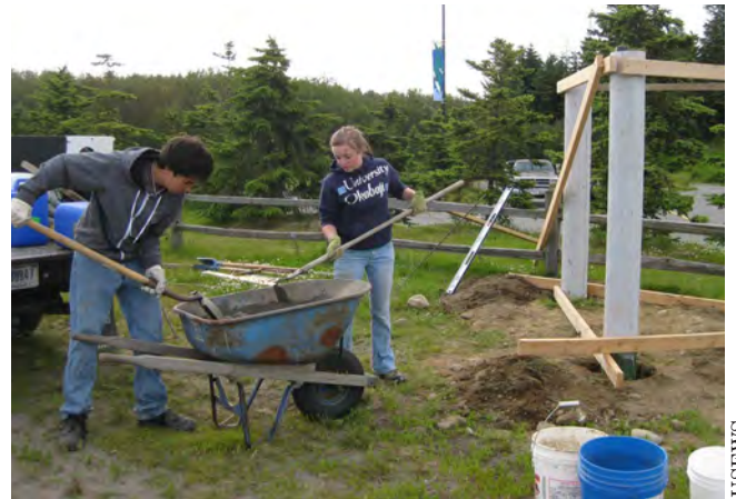
Ithaca and Traven working on sign posts.
