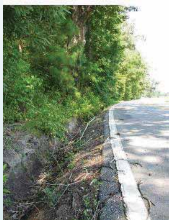
PHOTO SHOWS THE LACK OF A PAVED SHOULDER AND CLOSE PROXIMITY OF FIXED OBJECTS TO THE ROADWAY.
