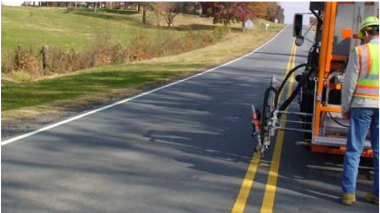
Figure 21. The cylinder can stretch 24 inches (0.6 meter) to adjust its installation position.
