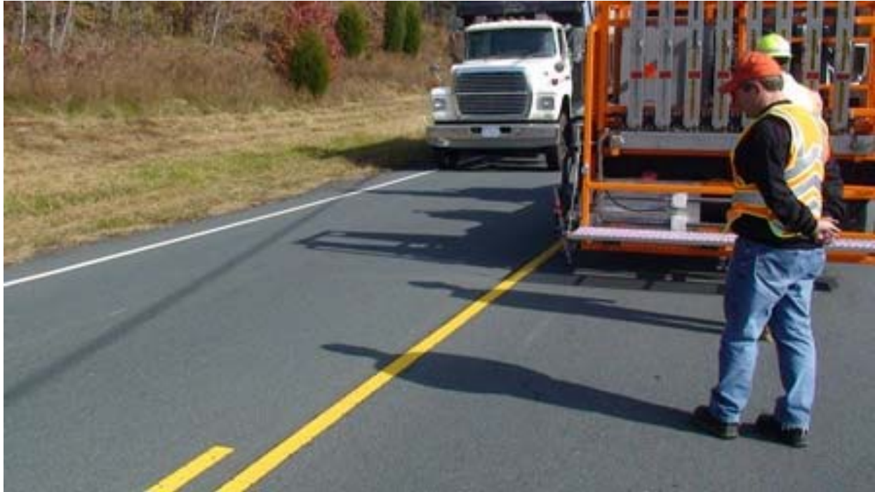
Figure 24. The robotic arm can be retracted when a large truck passes by to improve safety.
