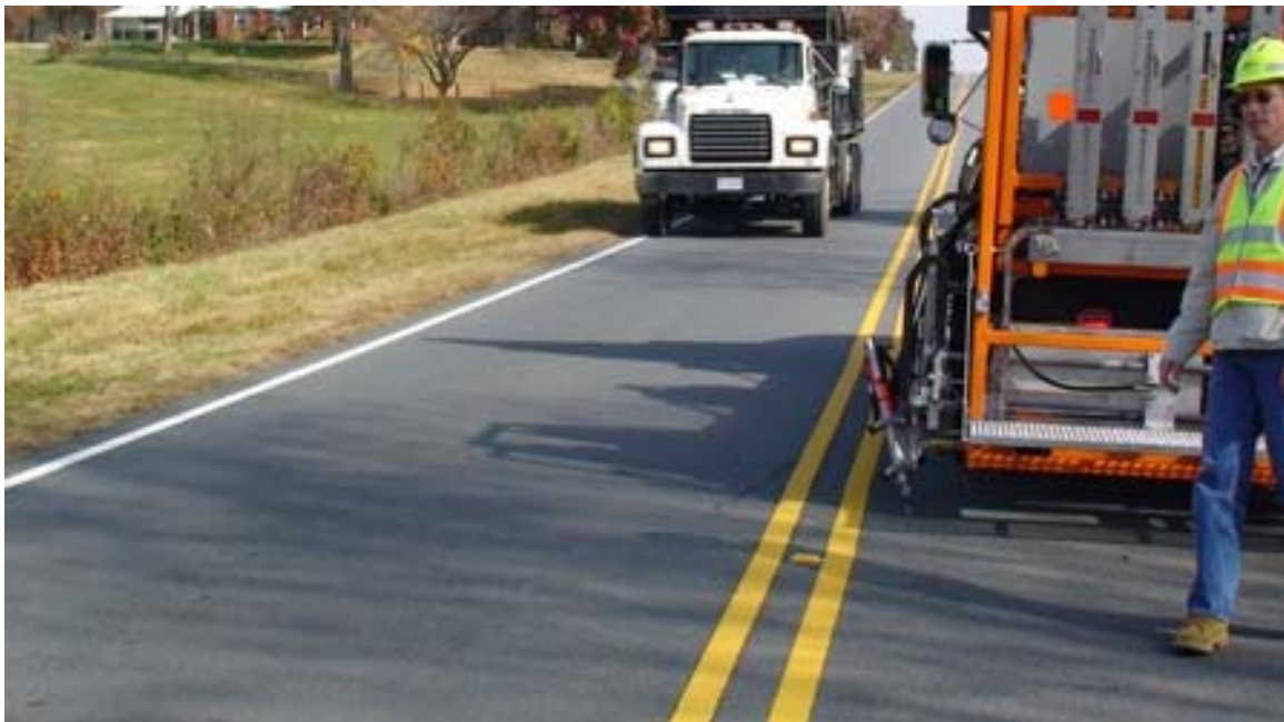
Figure 20. Installation operation under normal traffic conditions.
