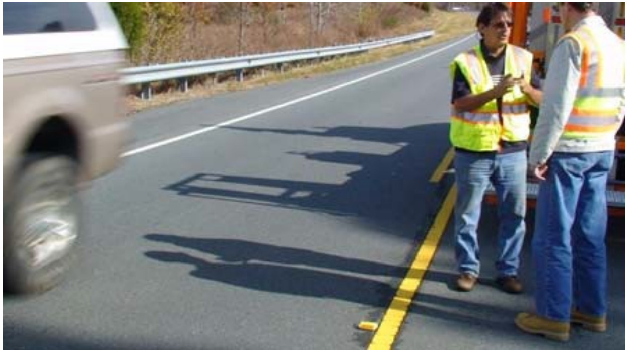
Figure 23. The installation quality could not be better, according to inspections.
