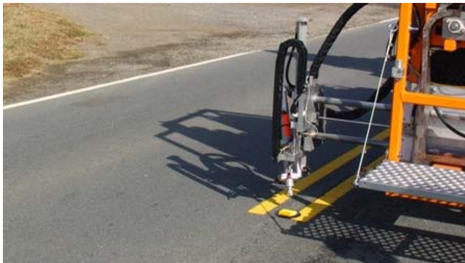
Figure 9. Delivery arm can stretch 24 inches (0.6 meter) to adjust its installation position.
