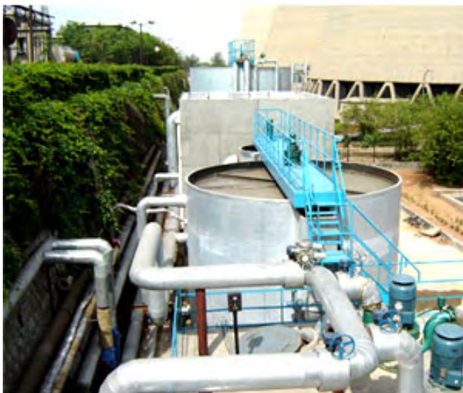
FIGURE 3.14 BAF SYSTEM AT A WWTP
