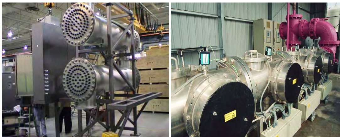
FIGURE 3.6 CLOSED-VESSEL UV REACTORS
