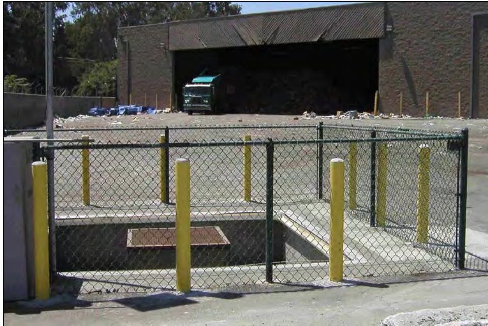
Figure 7 Sun Valley Recycling Facility Detention Basin
