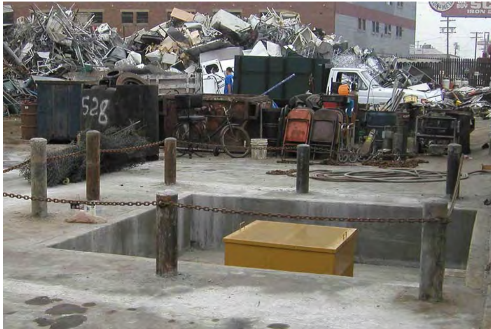
Figure 6 Metal Recycler Detention Basin
