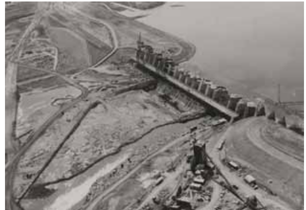
Pueblo Dam construction in the 1970s.
