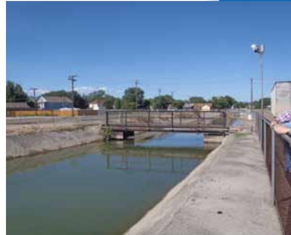
Pueblo Dam South Alternative alignment along Bessemer Ditch in Pueblo.
