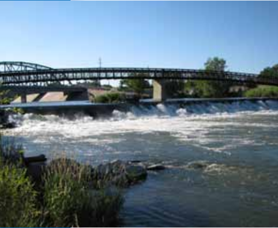
The River South Alternative river intake location would be near the Arkansas River at Moffat St. gage. A new diversion structure may be needed.
