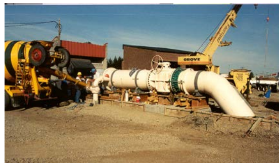
Photo 2-12. Pipeline appurtenances, such as valves, would be required along AVC.
