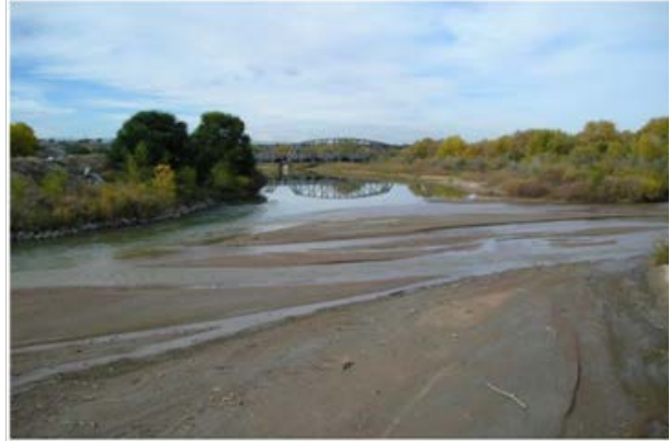
Source: Courtesy of U.S. Army Corps of Engineers Photo 3-12. Arkansas River at Fountain Creek confluence in 2009 (upstream view from the state Highway 227 bridge showing sediment deposition at the confluence).
