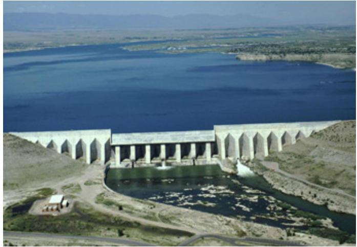
Photo 1-1. Pueblo Dam and Reservoir is the terminal storage facility of the Fry-Ark Project.
