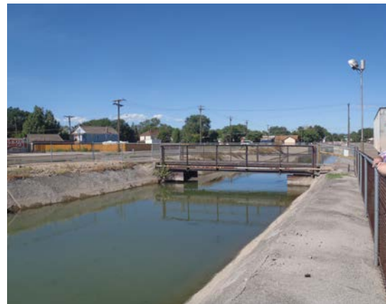
Photo 2-5. Pueblo Dam South Alternative alignment along Bessemer Ditch in Pueblo.
