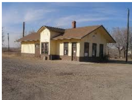
Photo 3-55. Boone Railroad Depot.
