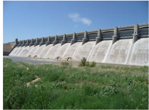
Photo 5-5. John Martin Dam
