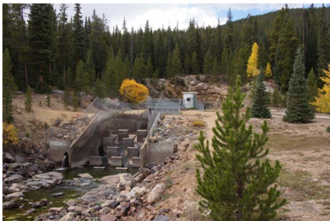
Photo 3-4. Boustead Tunnel outlet.
