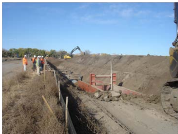
Photo 3-50. Typical pipeline construction activities.
