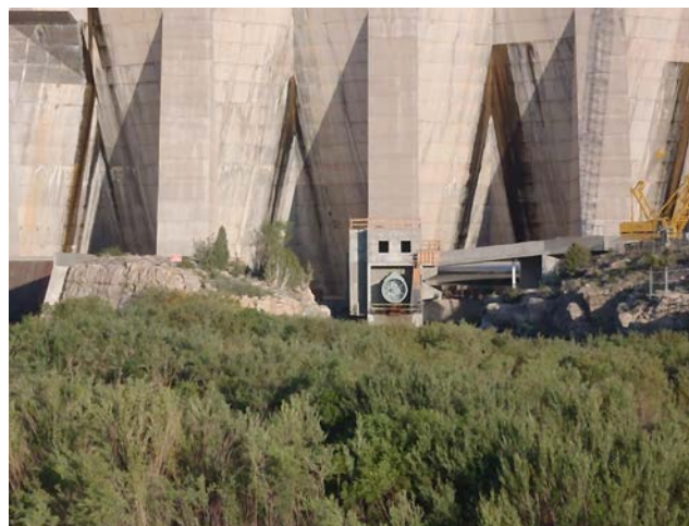
Photo 1-6. North Outlet Works and Southern Delivery System connection at Pueblo Dam.
