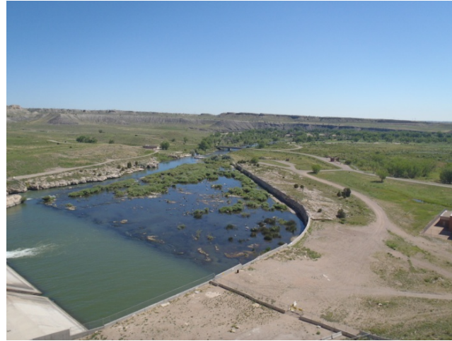
Photo 1-4. The Interconnect pipeline would connect the existing Pueblo Reservoir south outlet works manifold (bottom-right of photo, below ground) to the future north outlet works.
