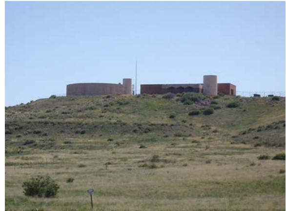
Photo 2-13. Water storage tanks, such as this tank on the existing Fountain Valley Conduit, would be used for operational storage and to provide a minimal amount of water if a system outage were to occur.
