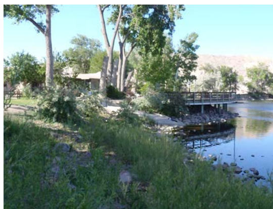
Photo 2-7. Pueblo Dam North Alternative alignment is near the Raptor and Nature Center of Pueblo, along the existing JUP.
