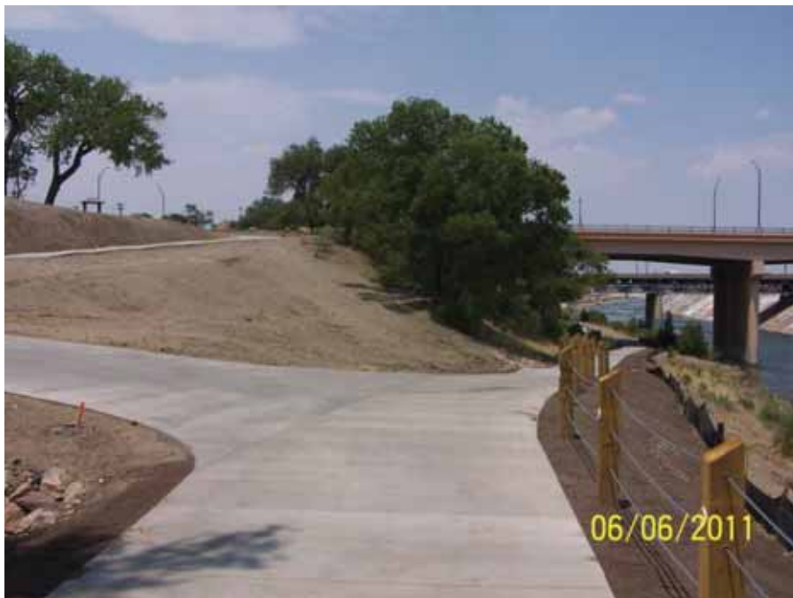
Photo 32 - AVC Alt 5 River South/North River Intake Pumping Plant site, looking west. Photo by Rodney Barthel
