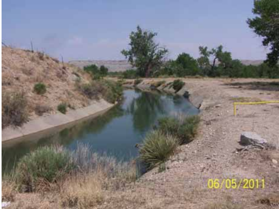
Photo 17 - Bessemer Ditch at Hwy 96 upstream, looking northeast. Photo by Rodney Barthel
