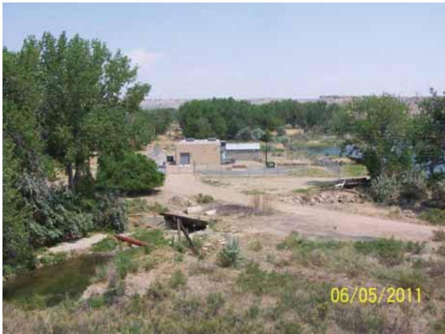
Photo 16 - BWWP Comanche Pump Station by Arkansas River. Photo taken looking north. Photo by Rodney Barthel
