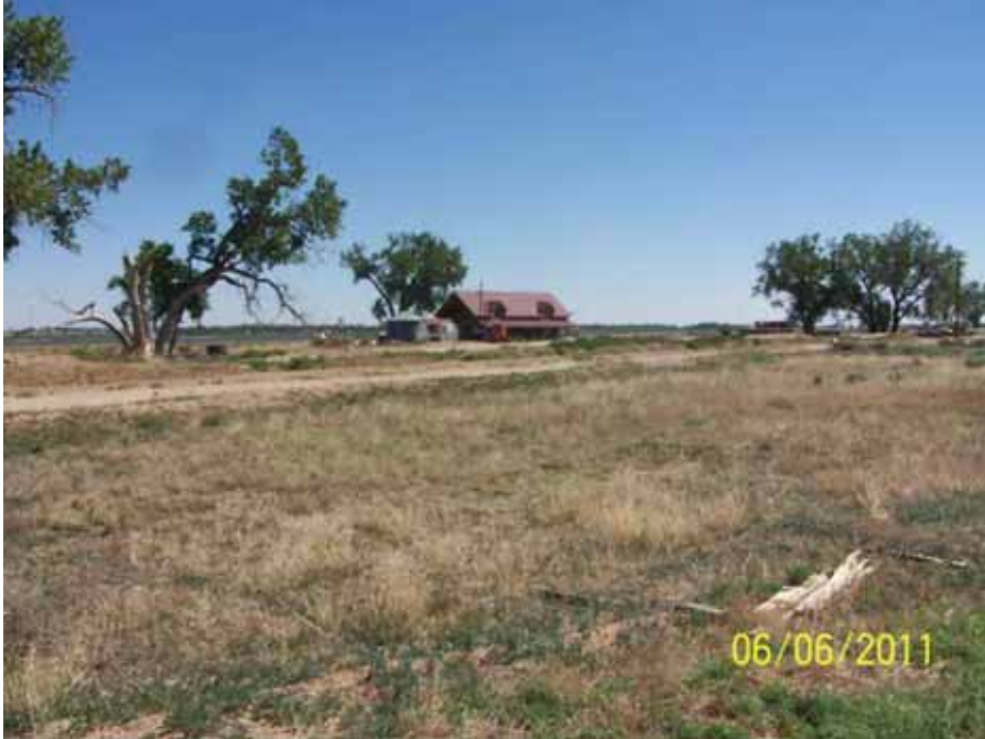
Photo 41 - AVC North La Junta Storage Tank site. Photo taken from Road 31, looking north. Photo by Rodney Barthel
