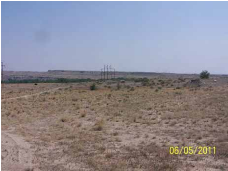
Photo 12 - AVC Alt 4 Pueblo Dam North WTP Site near BOR Field Office toward Pueblo Dam T-Lines. Photo by Rodney Barthel
