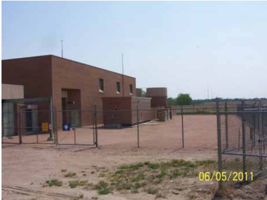
Photo 7 - Fountain Valley Authority Pump Station. Note unit substation located in front of building. Looking east. Photo by Rodney Barthel
