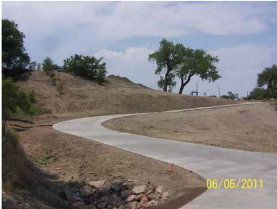
Photo 31 - AVC Alt 5 River South/North River Intake Pumping Plant site, looking west. Photo by Rodney Barthel
