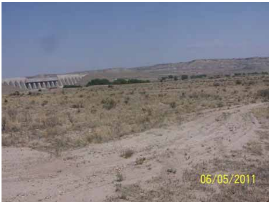
Photo 8 - AVC Alt 4 Pueblo Dam North WTP Site near Reclamation Field Office. Photo taken toward Pueblo Dam, looking northeast. Photo by Rodney Barthel
