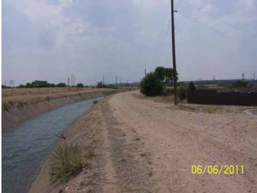
Photo 23 - AVC southern routes through Pueblo, behind (north east) of steel mill site by Bessemer Ditch, looking north. Photo by Rodney Barthel
