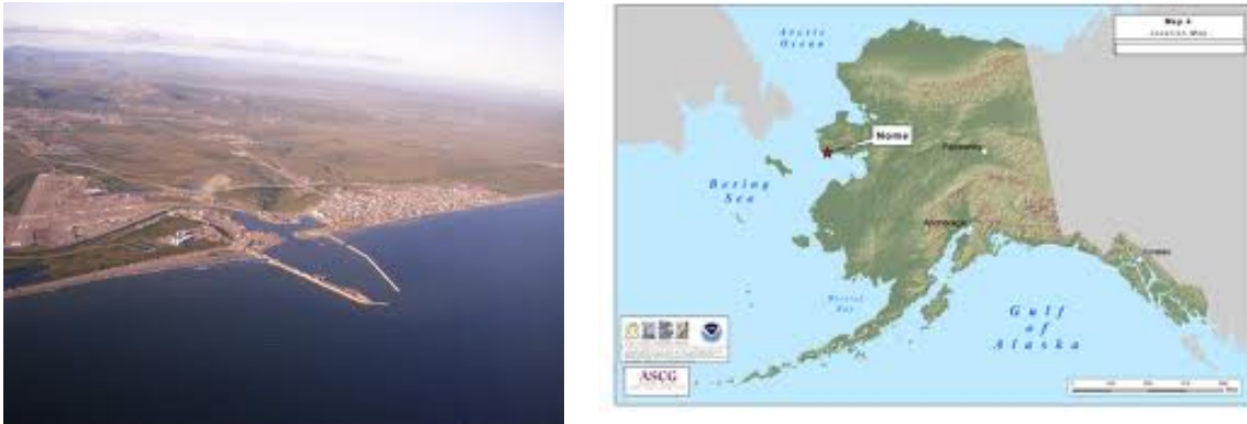
Figure 49: Port of Nome view (left). Nome location (right)
