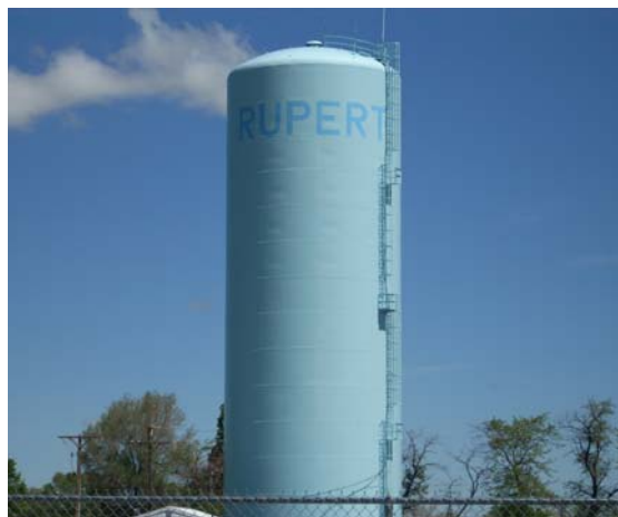
City of Rupert's 1.1 million gallon water storage tank. (EPA OIG photo)
