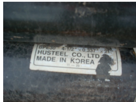
Grouting pipes labeled Made in Korea . (EPA OIG photo)
