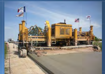
Including the Safety Edge SM in concrete slip-form paving requires a modified profile pan shape – no location specified for this one either
