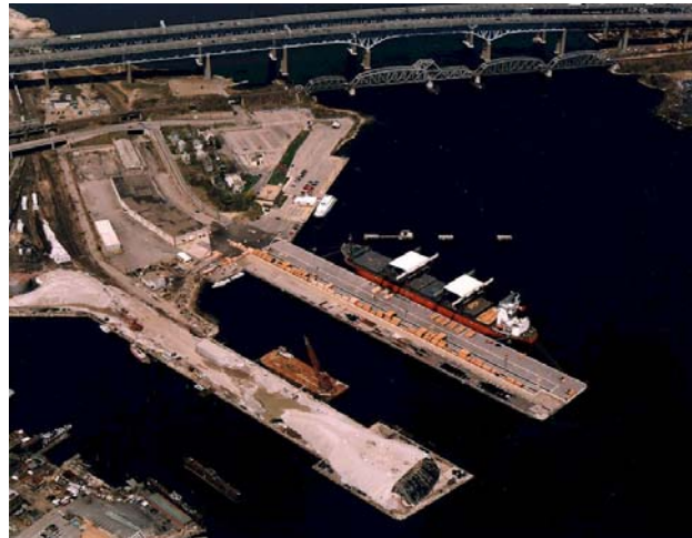
Picture Source: Connecticut Department of Transportation. 4
