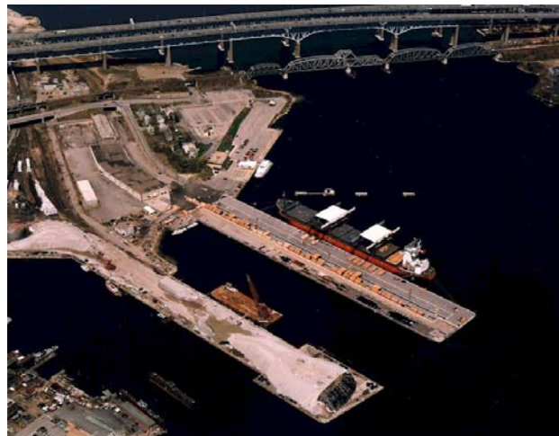
Picture Source: Connecticut Department of Transportation. 4
