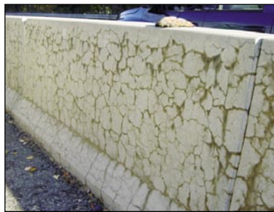
Figure 3. Concrete barriers along State Highway 2 near Leominster, MA.
