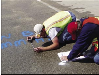
Figure 13. Expansion measurements being conducted after pavement was treated with lithium nitrate.
