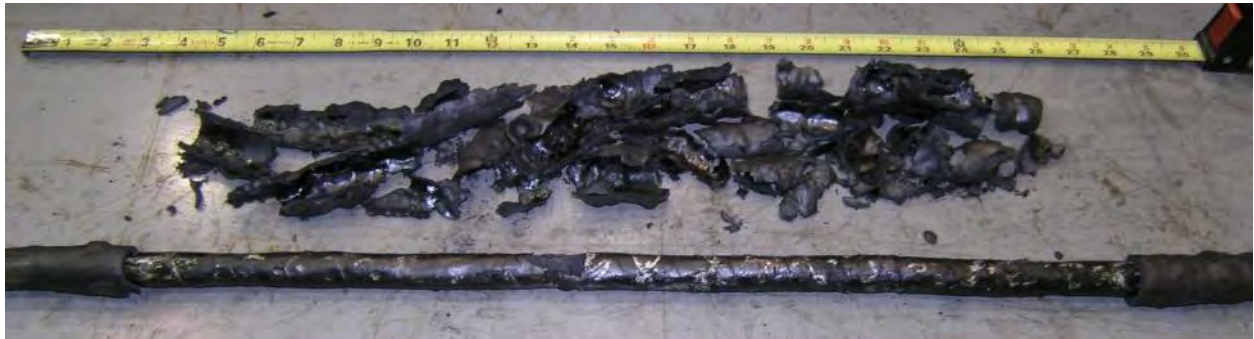
Figure 7.46: Jacketing material removed from the thermally exposed portion of the energized cable.
