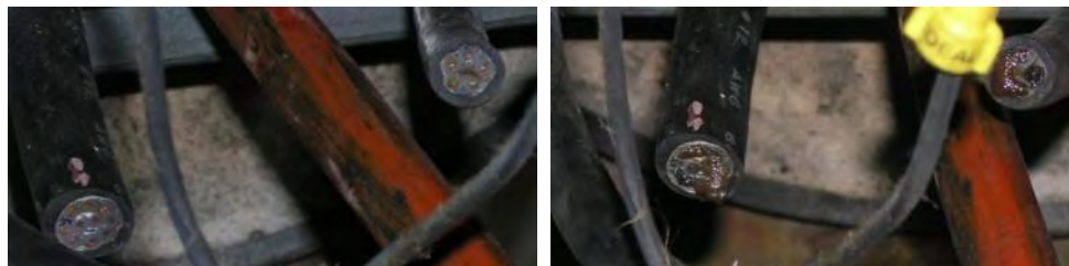
Figure 7.11: A pre-test view of the test cables (left) and a photo taken during the Test 15 (right) showing liquid leaking from the cut ends of the both of the thermal response cables (the 10/C and 5/C cables).
