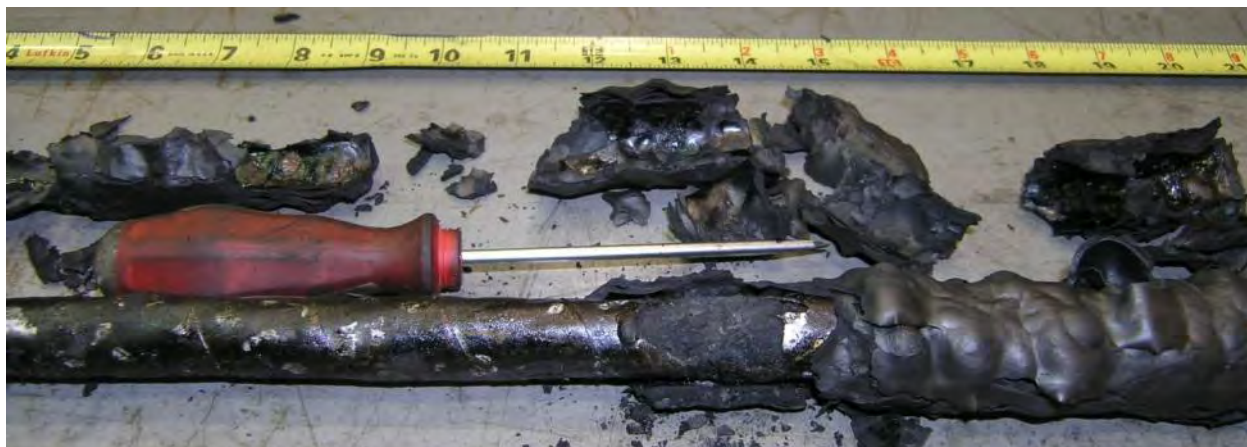
Figure 7.44: Large hole uncovered during the removal of the jacketing material.
