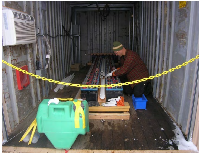
Figure A.12: Photo of the battery assembly.
