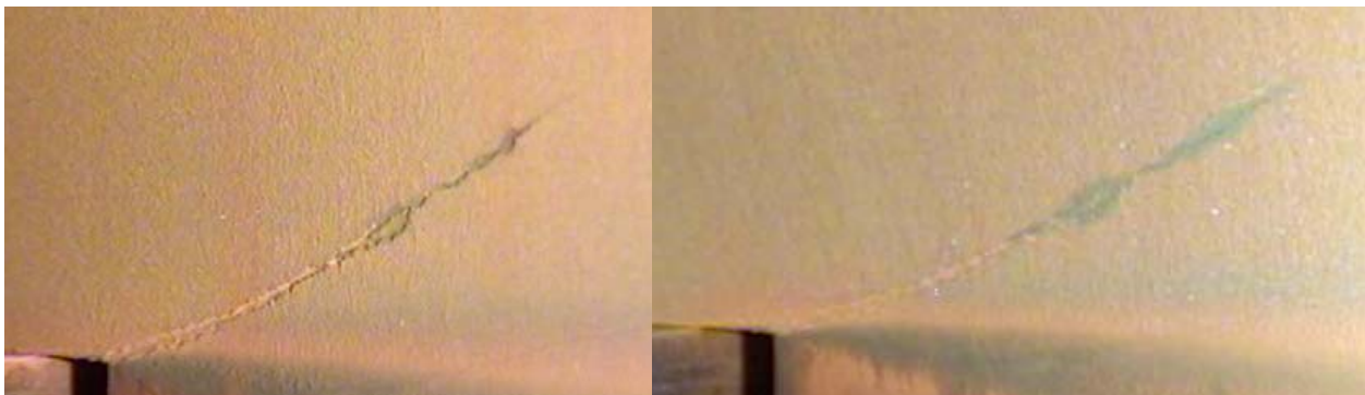
Figure 6.5 Mechanical Fatigue Crack Made Visible by Disturbance in Loose Oxide Layer
