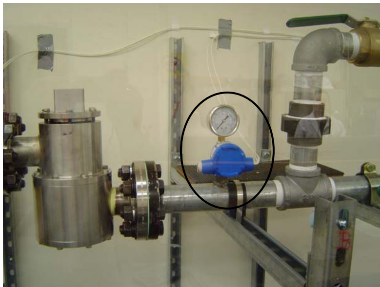
Figure 2-8. Detail Showing Location of Upstream Pressure Transducer
