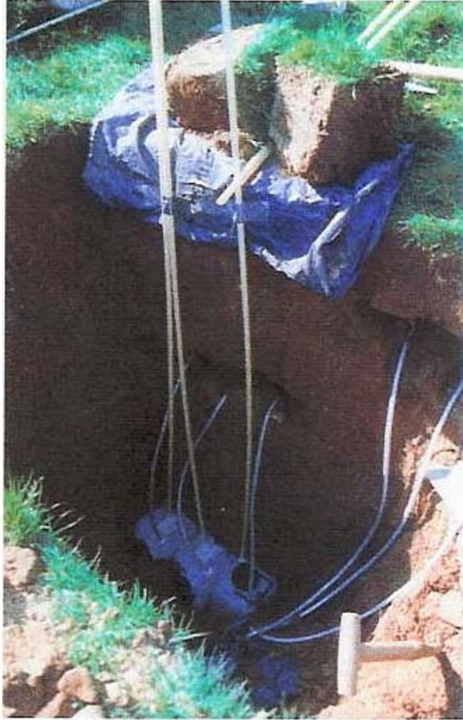
Figure 3-5. Installation of passive capillary samplers (after Jacques, 2000). With permission.
