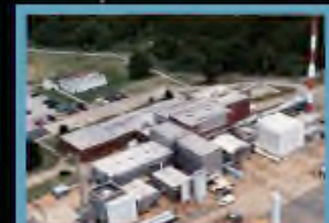
8-Ft High Temperature Tunnel Large-scale Hypersonics & Propulsion
