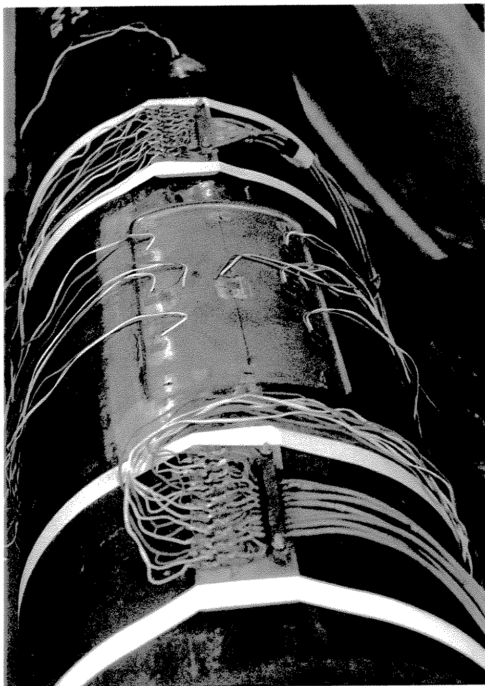
Figure 3-4 Picture of a corrosion defect with strain gauge instrumentation
