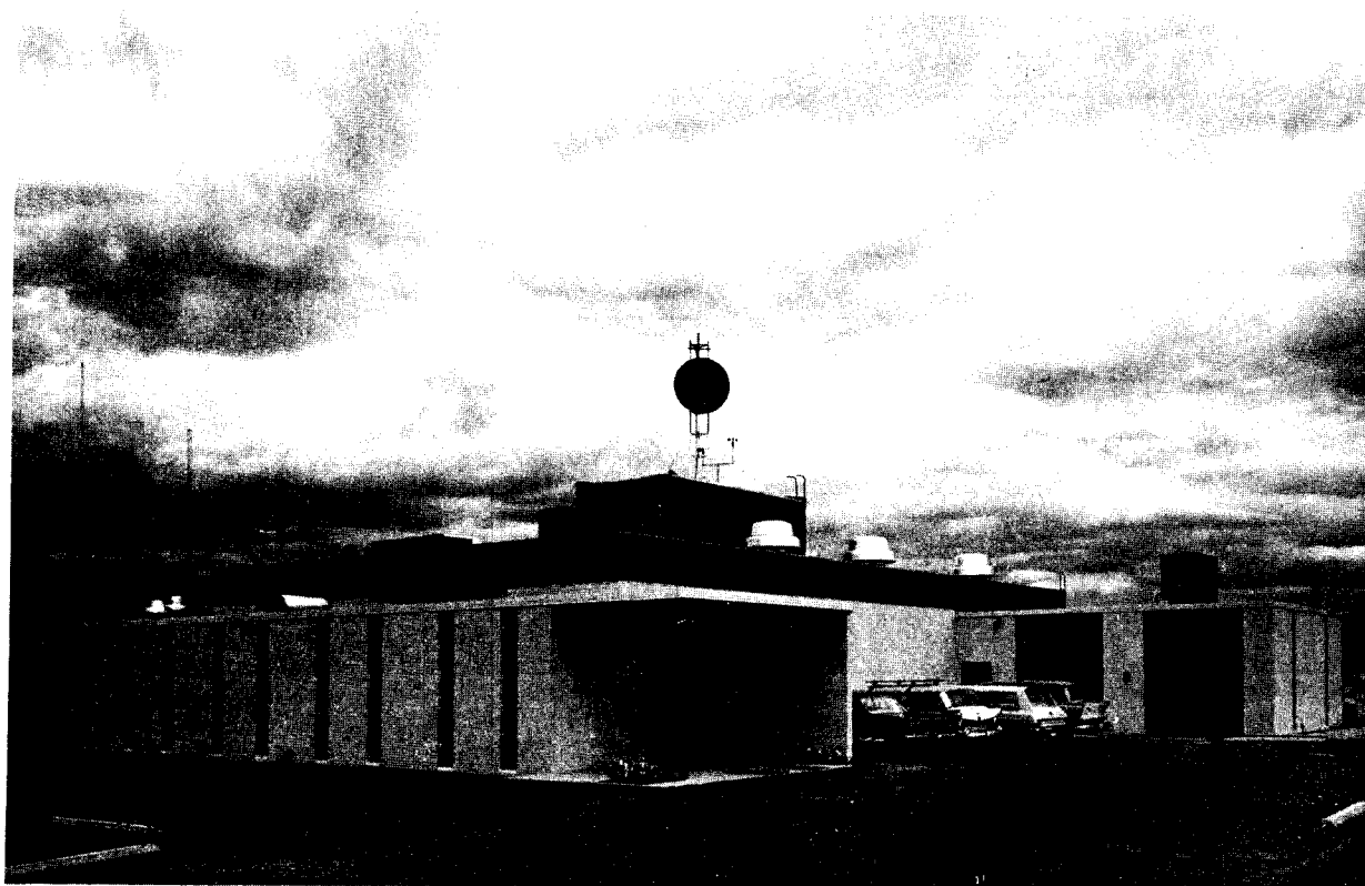
NBS Fort Collins facility showing WWV transmitter building.
