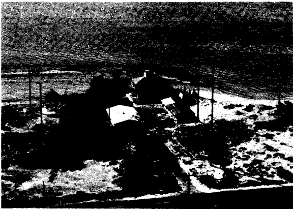
Antennas, transmitter building, and administrative buildings, WWVH, Maui, Hawaii.
