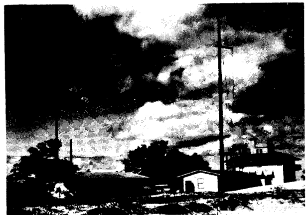
NBS Fort Collins facility in upper photo, showing the WWVB and WWVL transmitter building in the center, new 470-foot standby antenna mast in center, and 400-foot main masts on each side which are part of the two, four-mast antenna systems, WWVL to the left and WWVB to the right. At lower left are WWV transmitter building and antennas at Greenbelt, Maryland. At lower right are antennas, transmitter building, and administrative buildings for WWVH, Maui, Hawaii.
