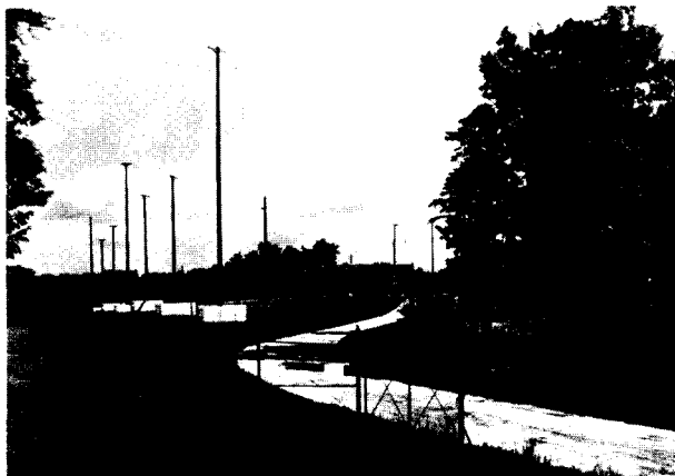
NBS Fort Collins facility in upper photo, showing the WWVB and WWVL transmitter building in the center, new 470-foot standby antenna mast in center, and 400-foot main masts on each side which are part of the two, four-mast antenna systems, WWVL to the left and WWVB to the right. At lower left are WWV transmitter building and antennas at Greenbelt, Maryland. At lower right are antennas, transmitter building, and administrative buildings for WWVH, Maui, Hawaii.
