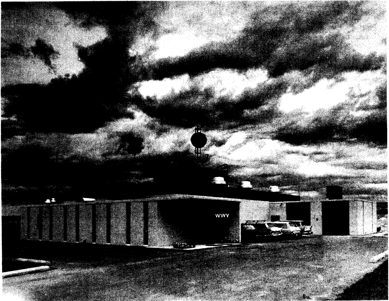
FIGURE 10.9. WWV transmitter building and antennas at Ft. Collins, CO.
