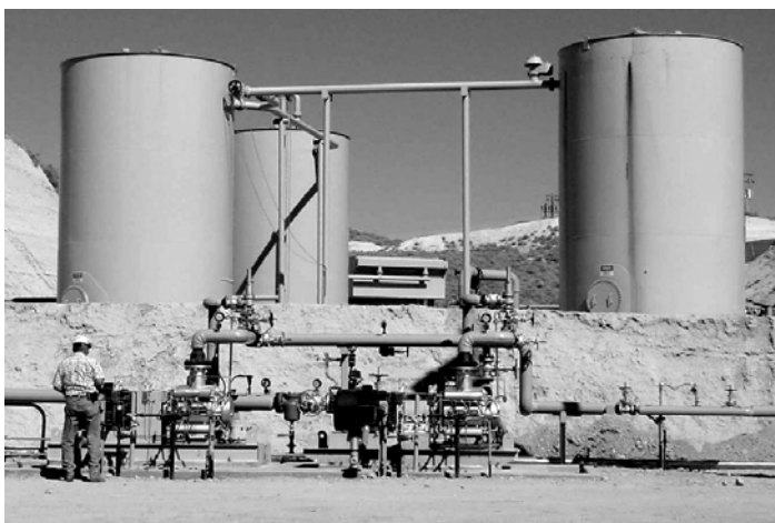
Figure. 9.4: Fin-fan cooler and progressive cavity pumps (a). Tanks and multiphase pumps (b).
