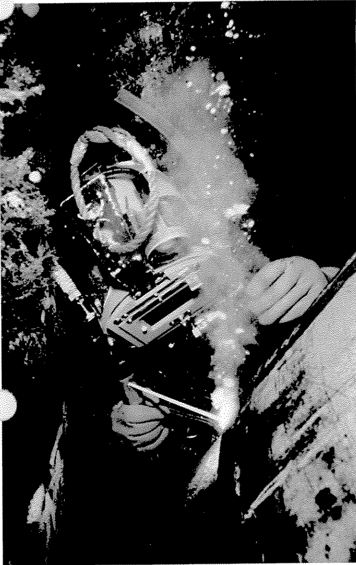
Welding With Global 1 Proprietary Electrodes
