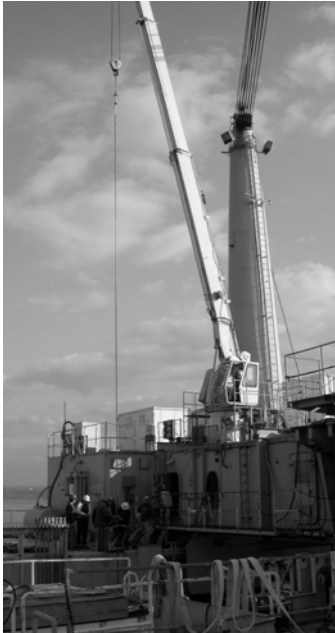
Pipe assembly with 80 foot capacity crane
