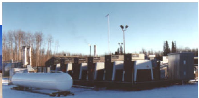
Mercury Electric's Numac Otter Installation
