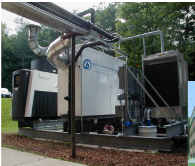
Microturbine/Absorption Chiller Integrated System at University of Maryland
