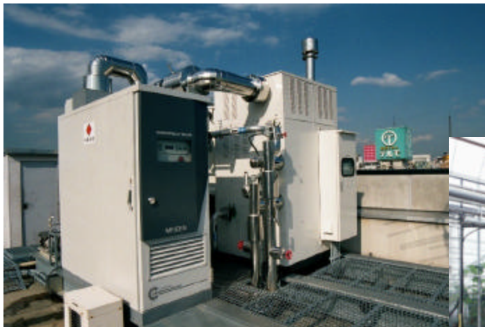
MEIDEN MioSpectrum Roof-Top Microturbine CHP Unit
