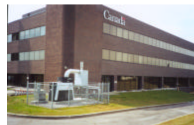
Midland Road Installation, Toronto
