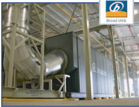
The IES includes a Broad absorption chiller rated at 2,535 refrigeration tons. The chiller produces 6,073 gpm of water chilled to 44°F.
