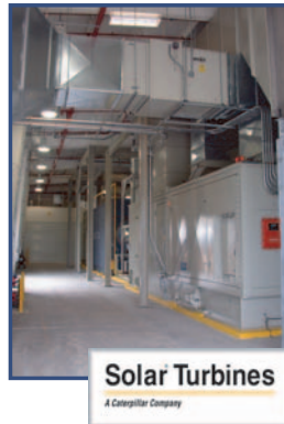
The IES includes a natural gas turbine and a heat-recovery chiller.
