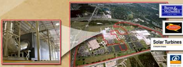
Turbine/Chiller System at Austin, Texas
