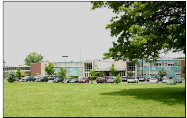
East Hartford High serves as an emergency shelter in its Connecticut community. The UTC Power PureComfort™ system provides power, cooling, and heating to the school.
