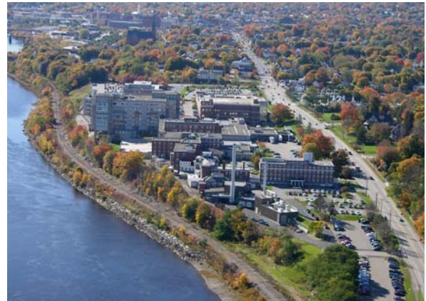
EMMC gets most of its electricity and steam from on-site combined heat and power installation
