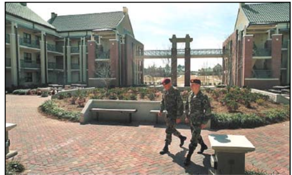
Turbine exhaust is used as a heat source for steam generation and a 1000-ton absorption chiller which produces chilled water that is used to condition barracks.
