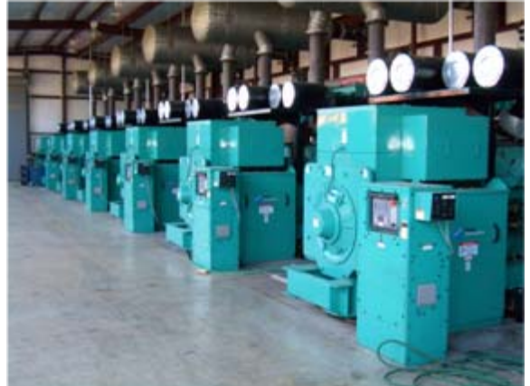
McMinnville Electric System's peaking power diesel generator sets
