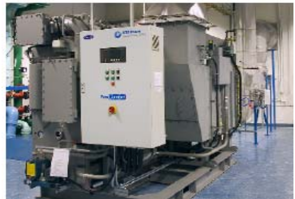
Lean-burn generator (above) and the absorption chiller/heater (below) are integrated to create the PureComfort Model 330R solution.
