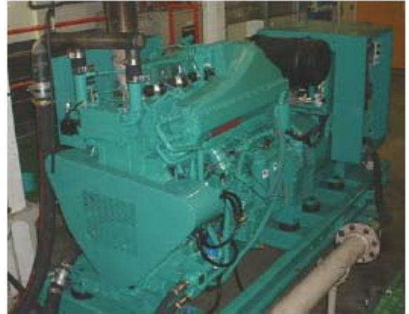
Lean-burn generator (above) and the absorption chiller/heater (below) are integrated to create the PureComfort Model 330R solution.
