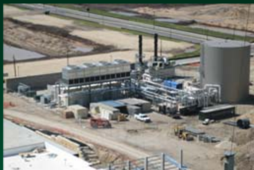
Packaged CHP system construction for the Dell Children's Medical District Energy System
