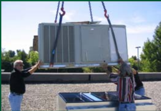
A conventional air-conditioning unit being installed on a standard curb mount fitted with the Trane CDQ™.
