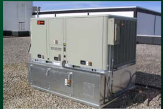
A conventional air-conditioning unit being installed on a standard curb mount fitted with the Trane CDQ™.
