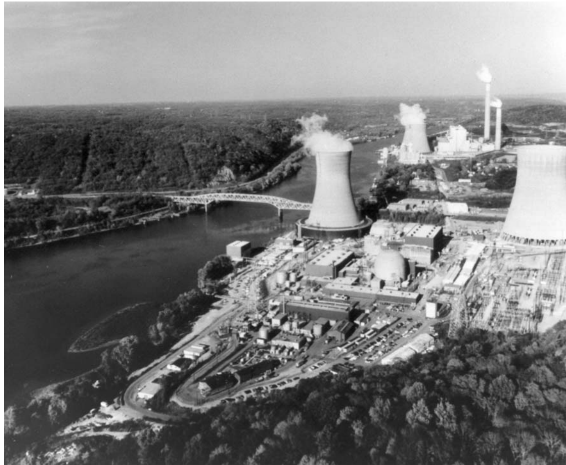
Site of Shippingport atomic power station, the first commercial nuclear power plant in the United States (rectangular reactor building and foreground); background, Beaver Valley 1 and 2 nuclear power plants and Bruce Mansfield coal-fired power plant (southwestern Pennsylvania). Source: U.S. Department of Energy.
