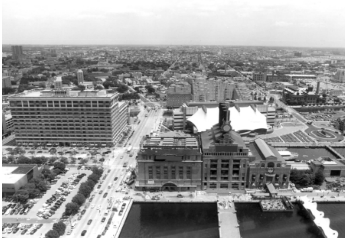
Office buildings, industries, residences, and transport systems, Baltimore, Maryland; east view from the Inner Harbor. Source: U.S. Department of Energy.
