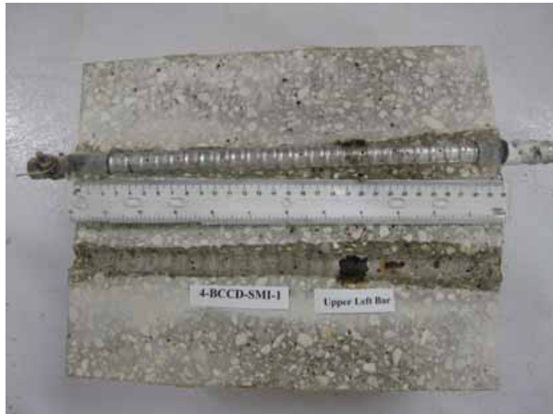
Figure 94. Photo. Top L bar and bar trace of specimen 4-BCCD-SMI-1 subsequent to dissection.
