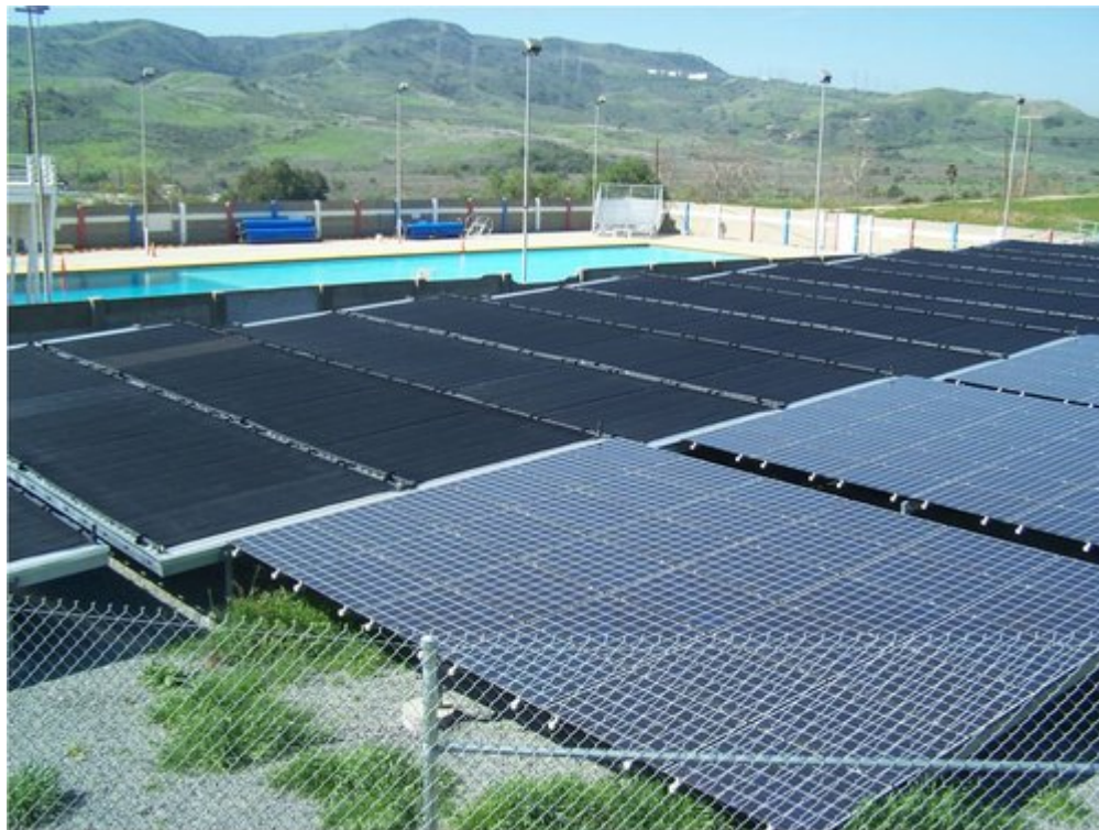
Figure 9: Solar pool heating system and solar photovoltaic system at Camp Pendleton, CA
