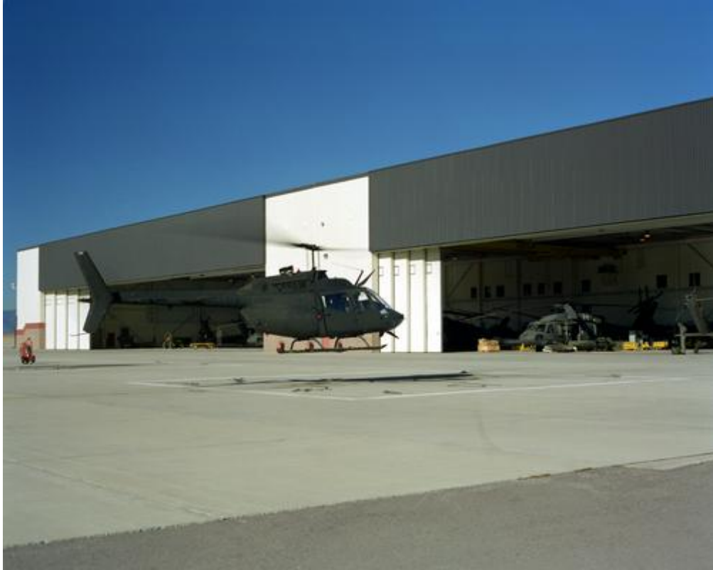
Figure 10: Solar ventilation preheating at Fort Carson, CO
