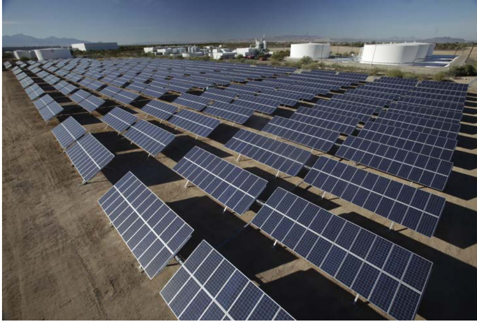
Photo from Marc Romito, Tucson Electric Power
